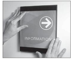
**3.** Align sign to level line. Apply pressure along tape line to activate pressure sensitive adhesive.
