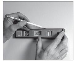
**1.** Draw a level line and wipe mounting surface clean of dust or debris.
