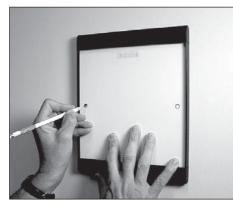
**1.** Draw a level line; align sign to this line. Transfer mounting hole pattern to wall
